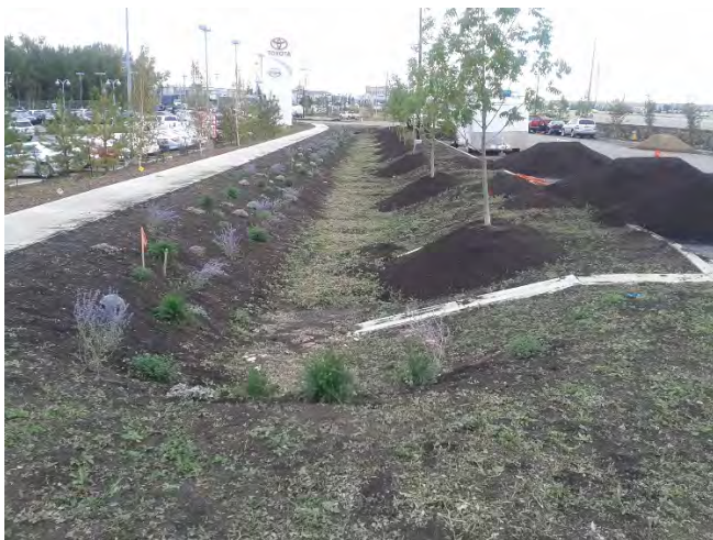
Bio-swale under construction
